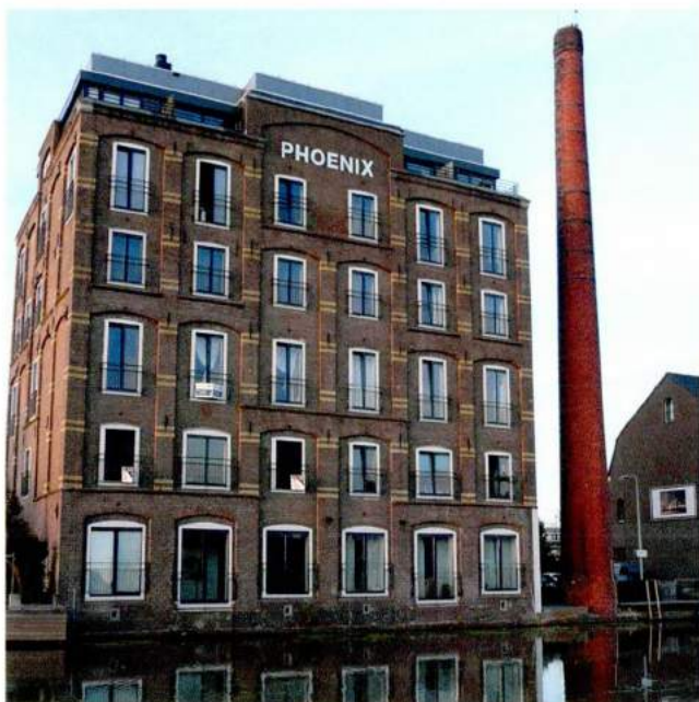
Appartementencomplex Phoenix te Bodegraven.
